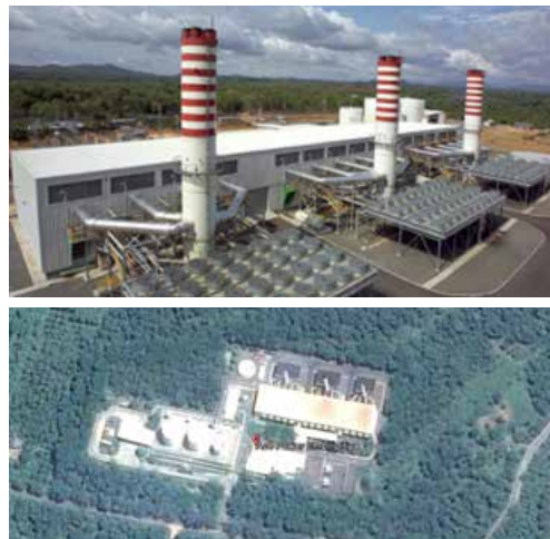
Figure 5.13 : ACE Power Plant Source : goo.gl/3kc6Q9
