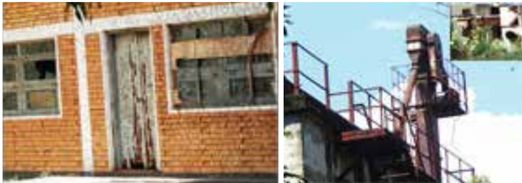
Figure 3.2 : Moraketiya Paddy Warehouse scheme Source : Local News, 2016
